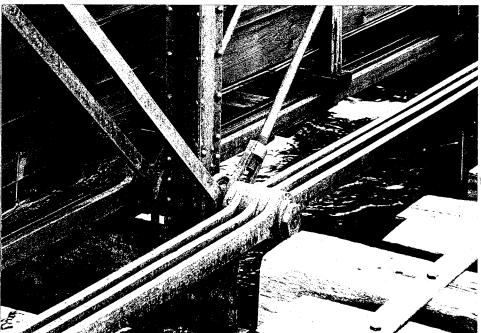
PHOTO # 12 Subject: Whipple Truss Bridge Berlin Mills Railway, BERLIN Detail of lower pin connection Photographer facing: NE Roll # 2 Frame # 16
